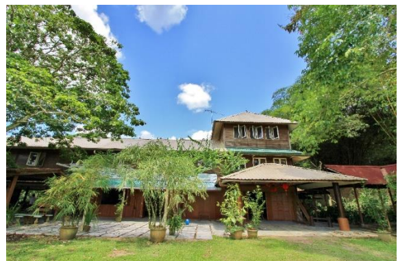
The wood lodge is the main building of TITI Eco Farm Resort.
